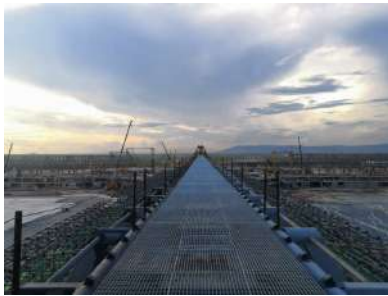
Steel grating maintenance
