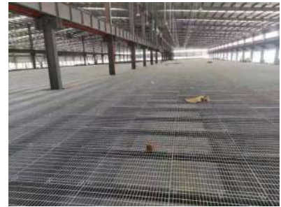
Steel grating logistics
