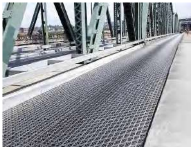
Steel grating bridge decks
